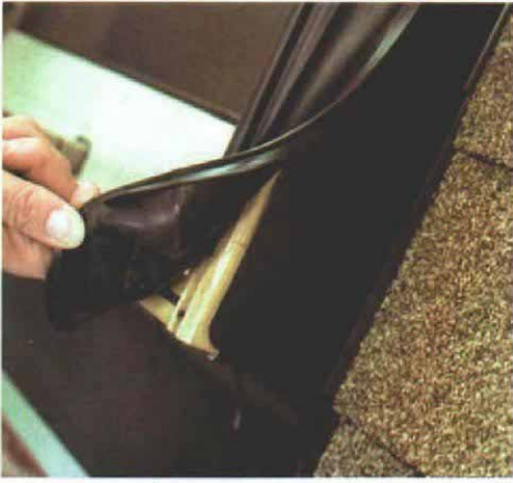
A rubber gasket seals the flashing. Many skylight manufacturers use rubber gaskets to cover the top of the flashing, such as the Roto skylight pictured here.
