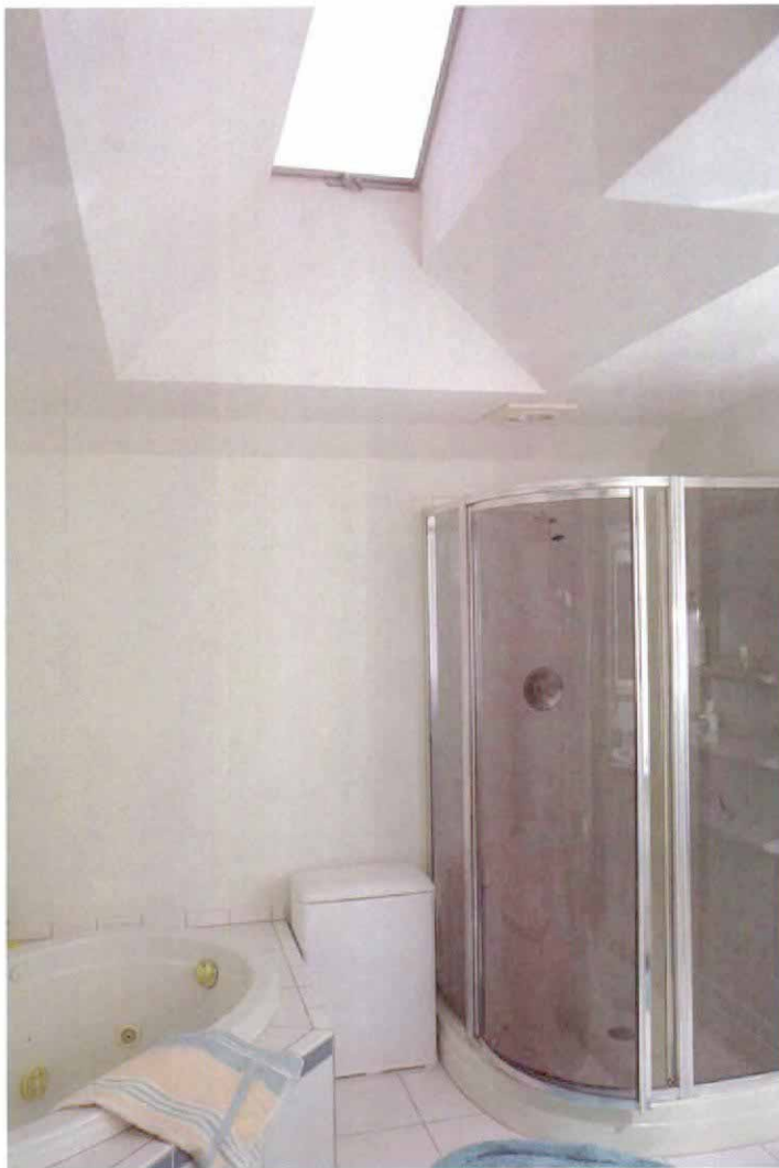
A skylight expands a bathroom. The splayed chase for this skylight not only lets in more light but also makes the bathroom feel roomier. Even though the bathroom is equipped with a powerful exhaust fan, an open skylight can provide a quick escape route for the warm, moist air from the shower and the spa.
