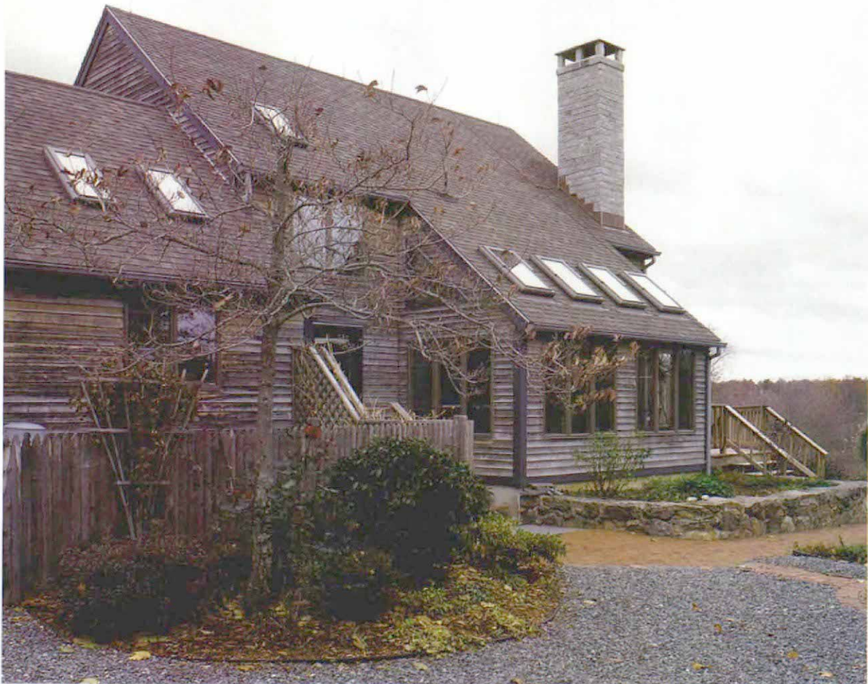
Skylights for different purposes. Skylights on the outside of this house punctuate the various roof planes. Inside, they serve a variety of functions, from kitchen light and ventilation, to ventilation and added views for a second-floor bedroom, to concentrated light and solar gain in the sunroom.
